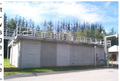
Blowing Rock Wastewater Plant
